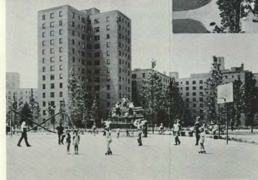
Older children find full opportunity for recreation with members of the PARKCHESTER staff cooperating. This is one of the Play Areas in the South Section.
