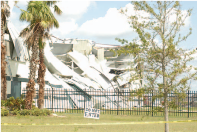
Florida building damaged by Hurricane Charlie.
