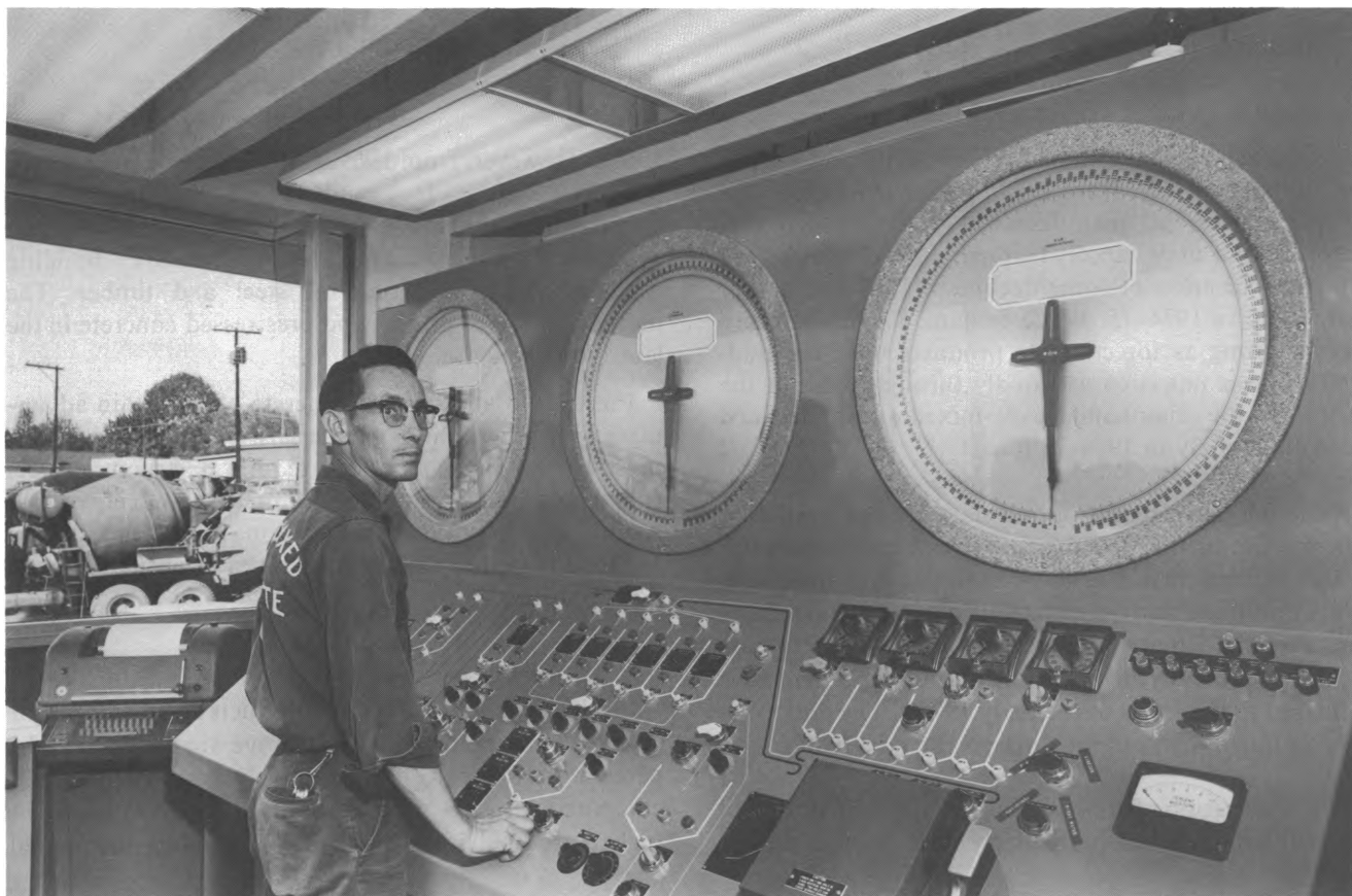
Automatic batching in which aggregates and cement are automatically selected and weighed to meet required specification.
