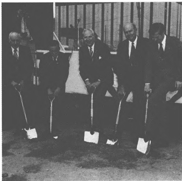
Officials of the Federal Reserve Bank of Richmond broke ground on April 18, 1975, for new Bank building on property overlooking the James River in the Main-to-the-James development area. Pictured from left to right are George C. Rankin, First Vice President, Robert P. Black, President, Robert W. Lawson, Jr., Chairman of the Board, E. Craig Wall, Sr., Deputy Chairman of the Board, and Richmond City Mayor, Thomas J. Bliley, Jr.
