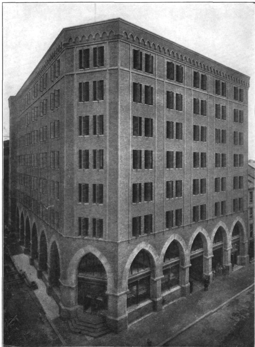
New Storage Building under erection at Maiden Lane and Gold Street
